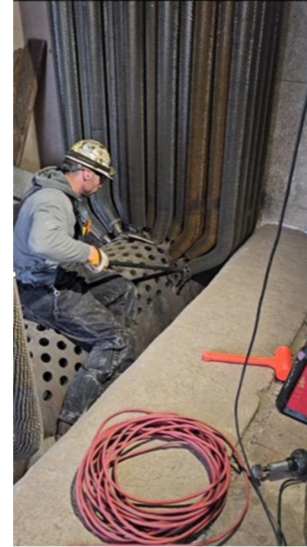
Replacing all 469 tubes
